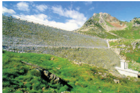
Escoubous dam (downstream view)
